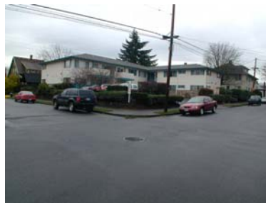
10/09 Sale- $92,500/Unit 10 unit Weidler Place Apartments 2624-2644 NE Weidler Street
